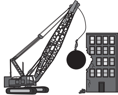
Wrecking ball breaking down a building
