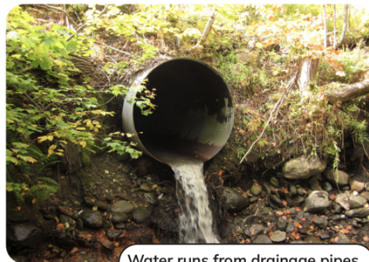
Water runs from drainage pipes into a creek.
