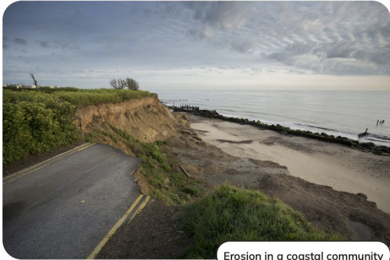
Erosion in a coastal community
